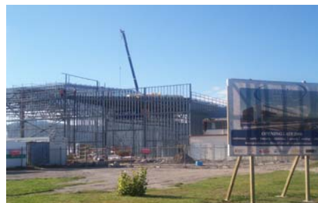
Work is progressing well at the new Energy Events Centre
